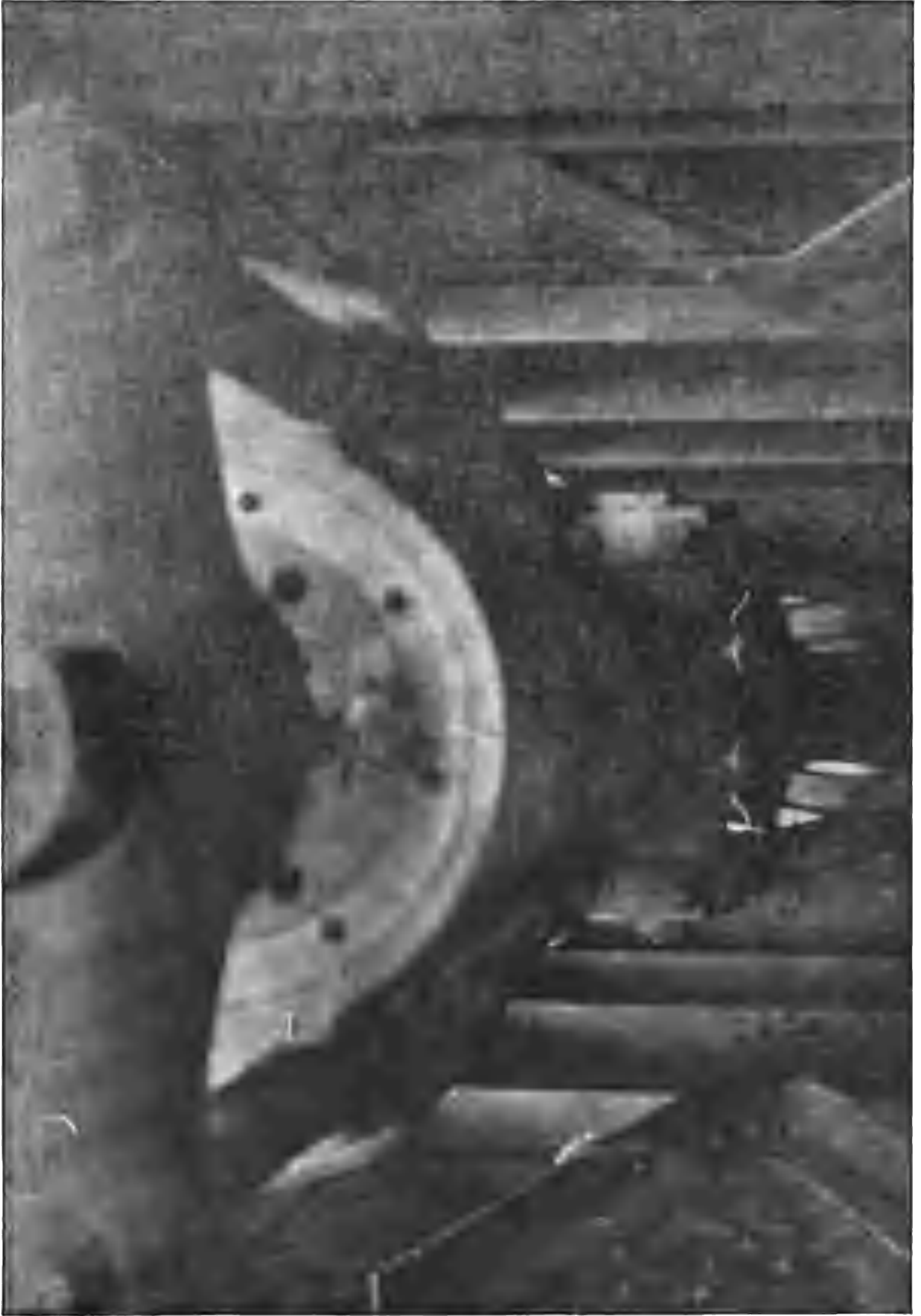
RECUPERATOR CYLINDER OF THE 390-MM. GERMAN GUN MOUNT.
