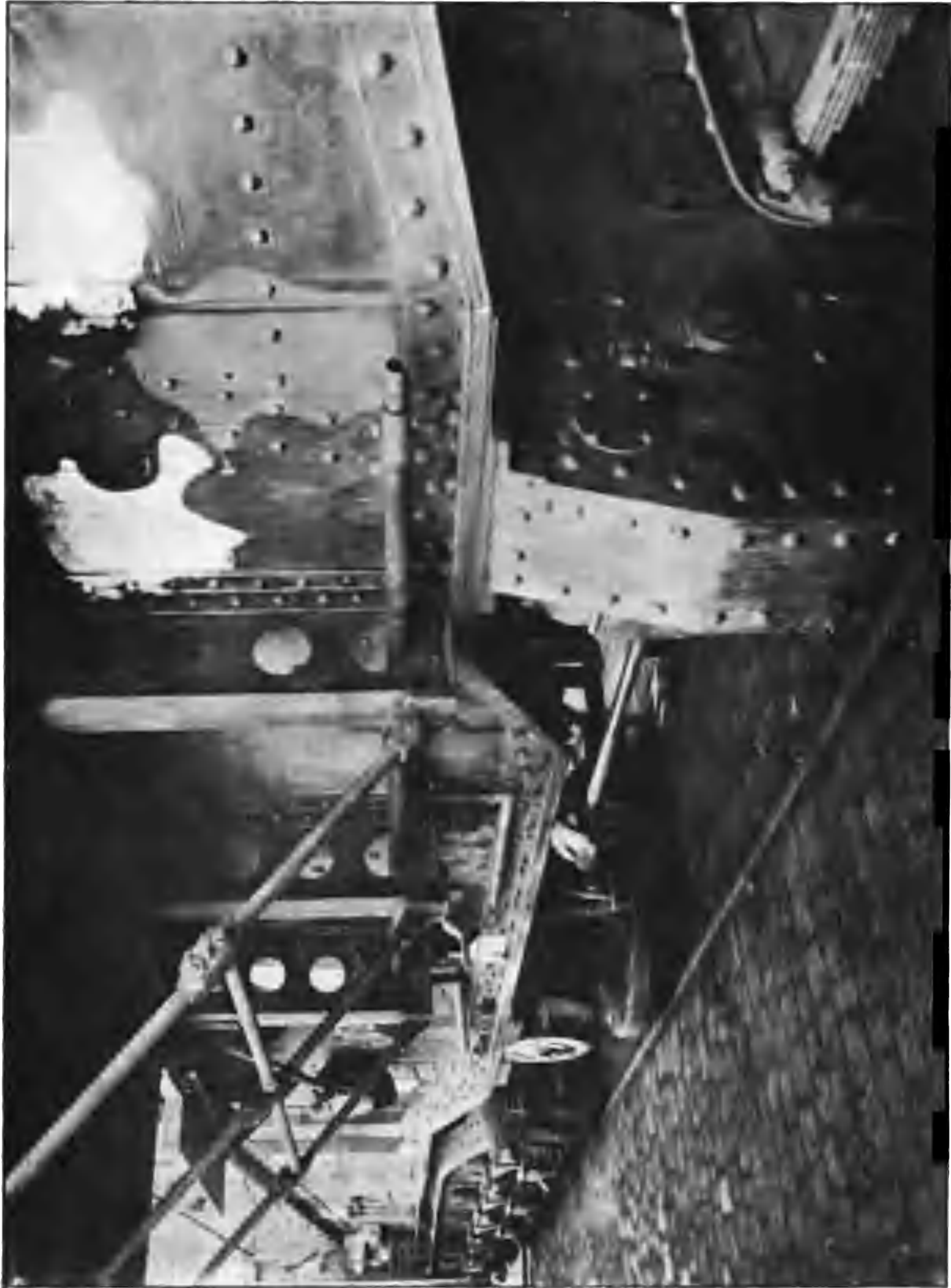
CENTER PIVOT AND TRAVERSING MECHANISM OF THE 280-MM. GERMAN GUN MOUNT.
