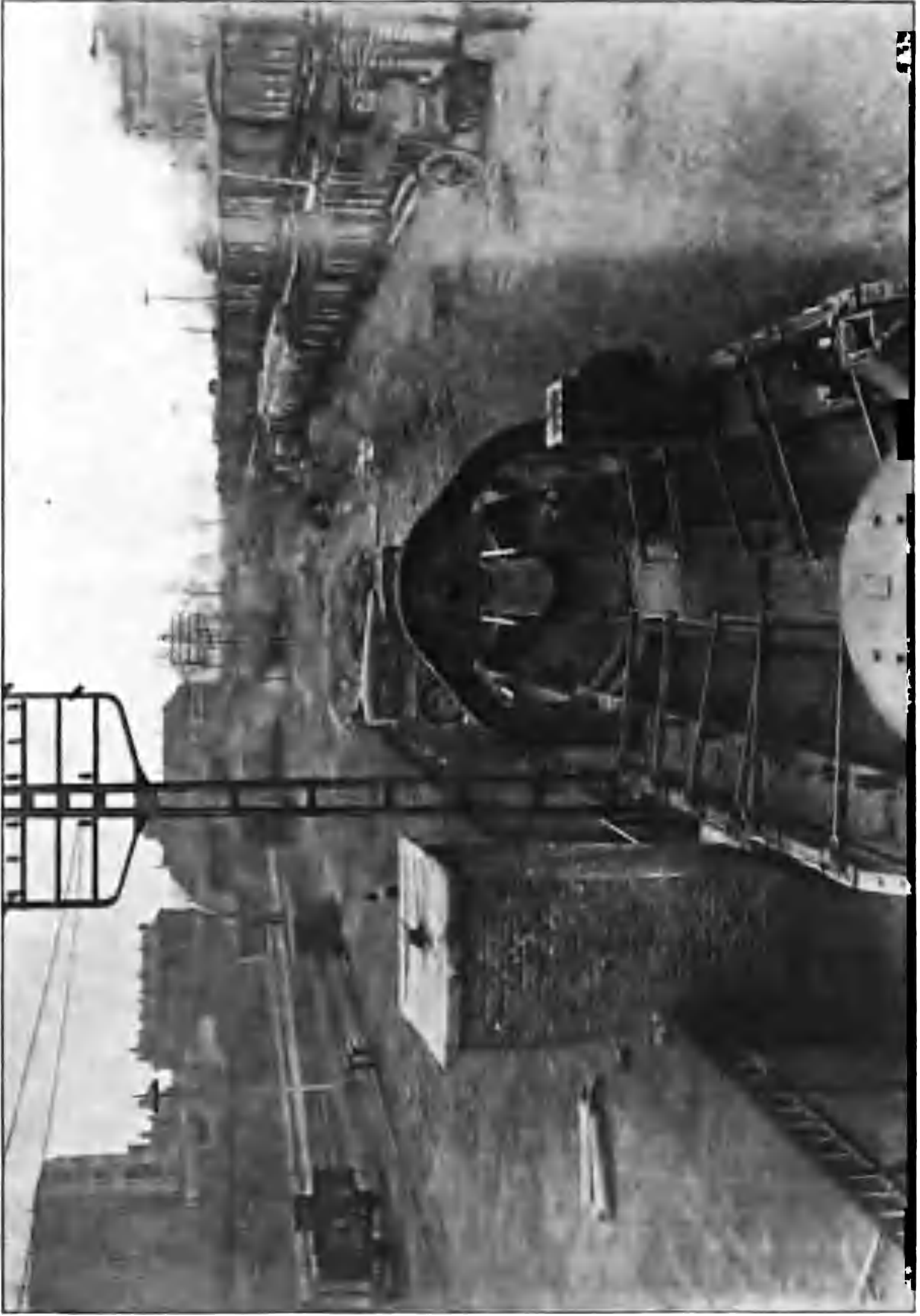
OPERATING PLATFORM, SHOT TRUCK, AND AMMUNITION HOIST OF THE 380-MM. GERMAN GUN MOUNT.
