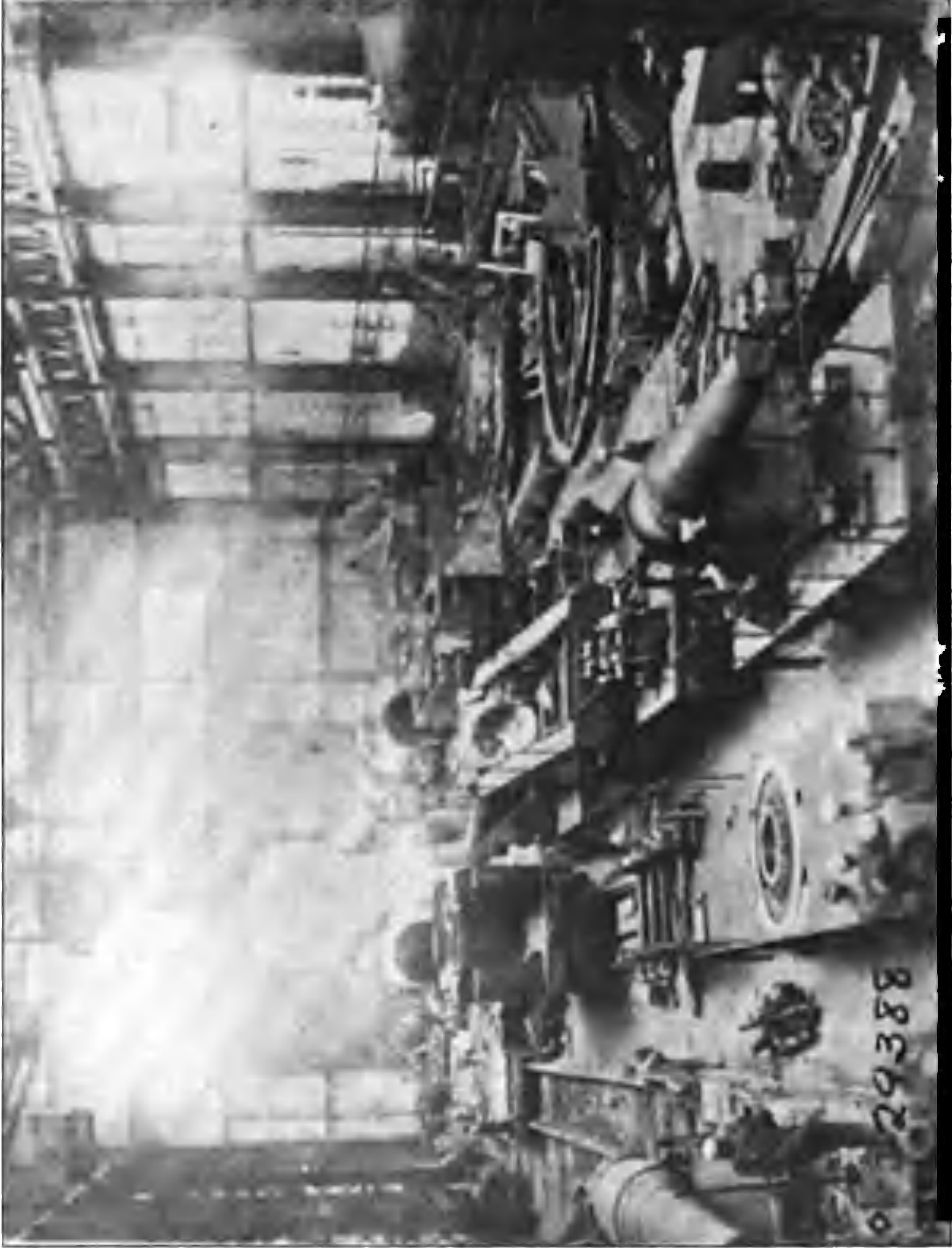
14-INCH, 50-CALIBER AMERICAN NAVY GUN MOUNT, MARK I, IN COURSE OF ERECTION IN THE CHANTIERS DE LA LOIRE ST. NAZAIRE, FRANCE.
