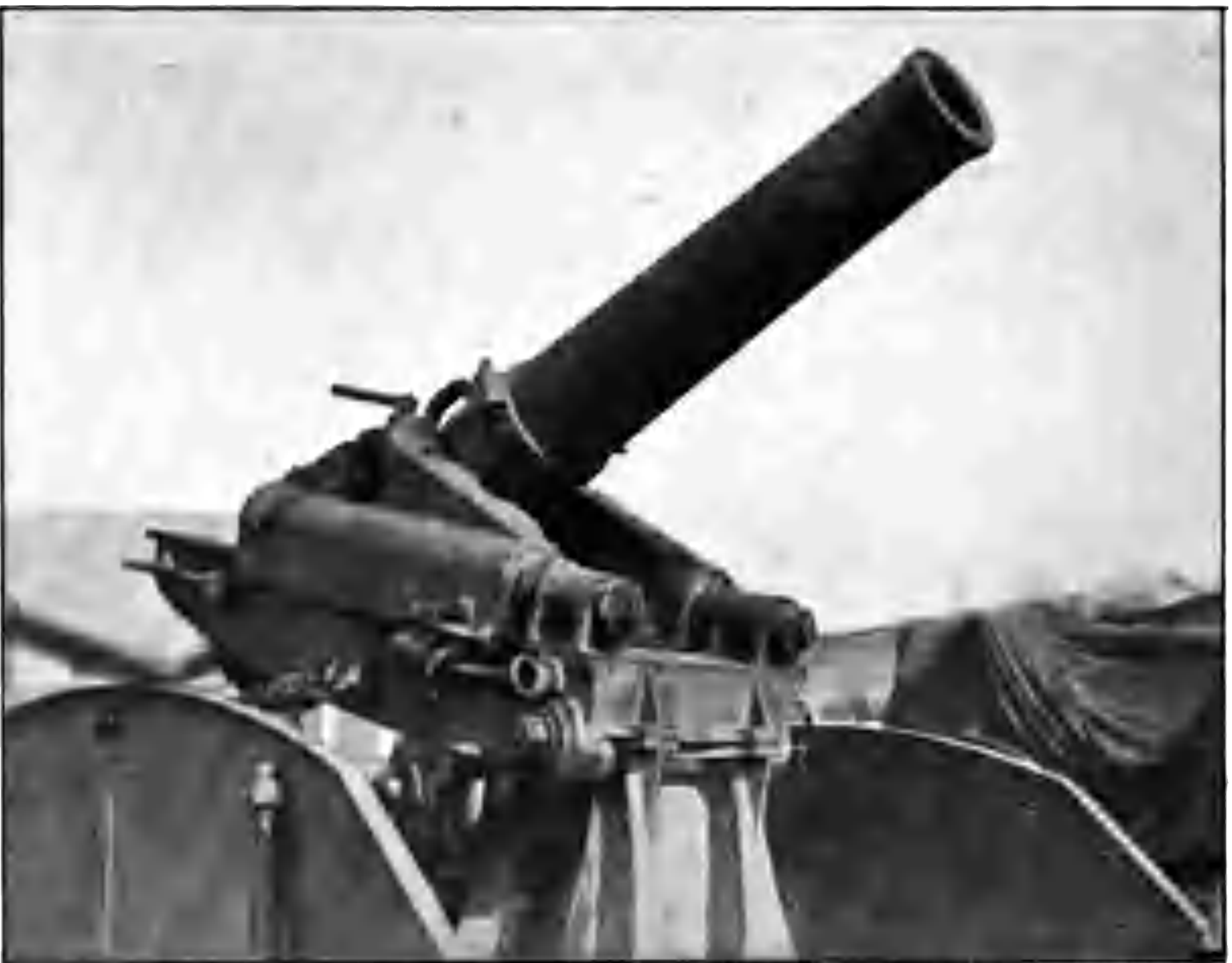
GUN CARRIAGE OF 155 MM. HOWITZER ON RAILWAY MOUNT.
