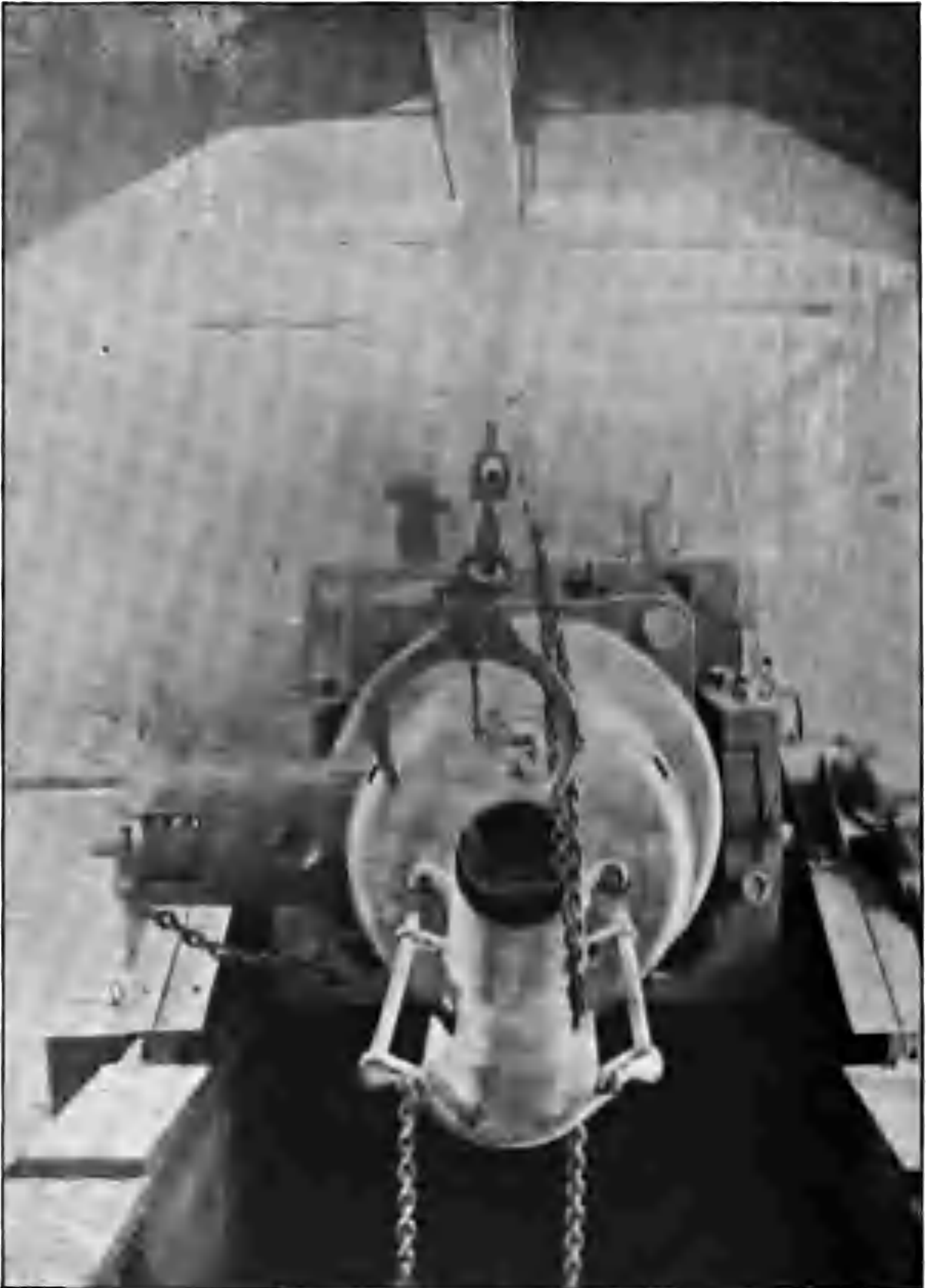
BREECH, CRADLE, AND LOADING TRAY OF THE 240-MM. GERMAN HOWITZER.
