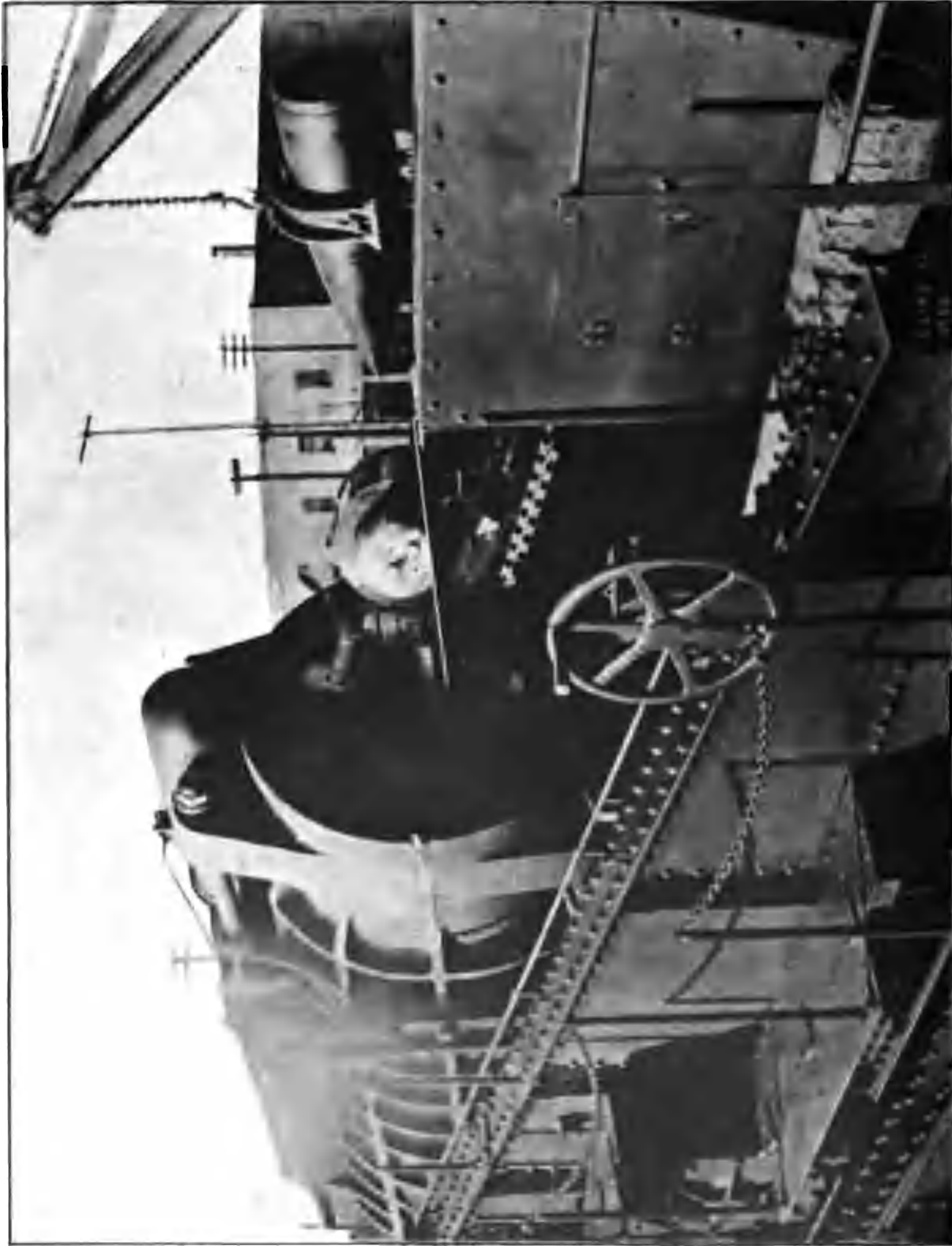
LOADING TABLE AND TRAY OF THE 12-INCH, 35-CALIBER AMERICAN GUN MOUNT.
