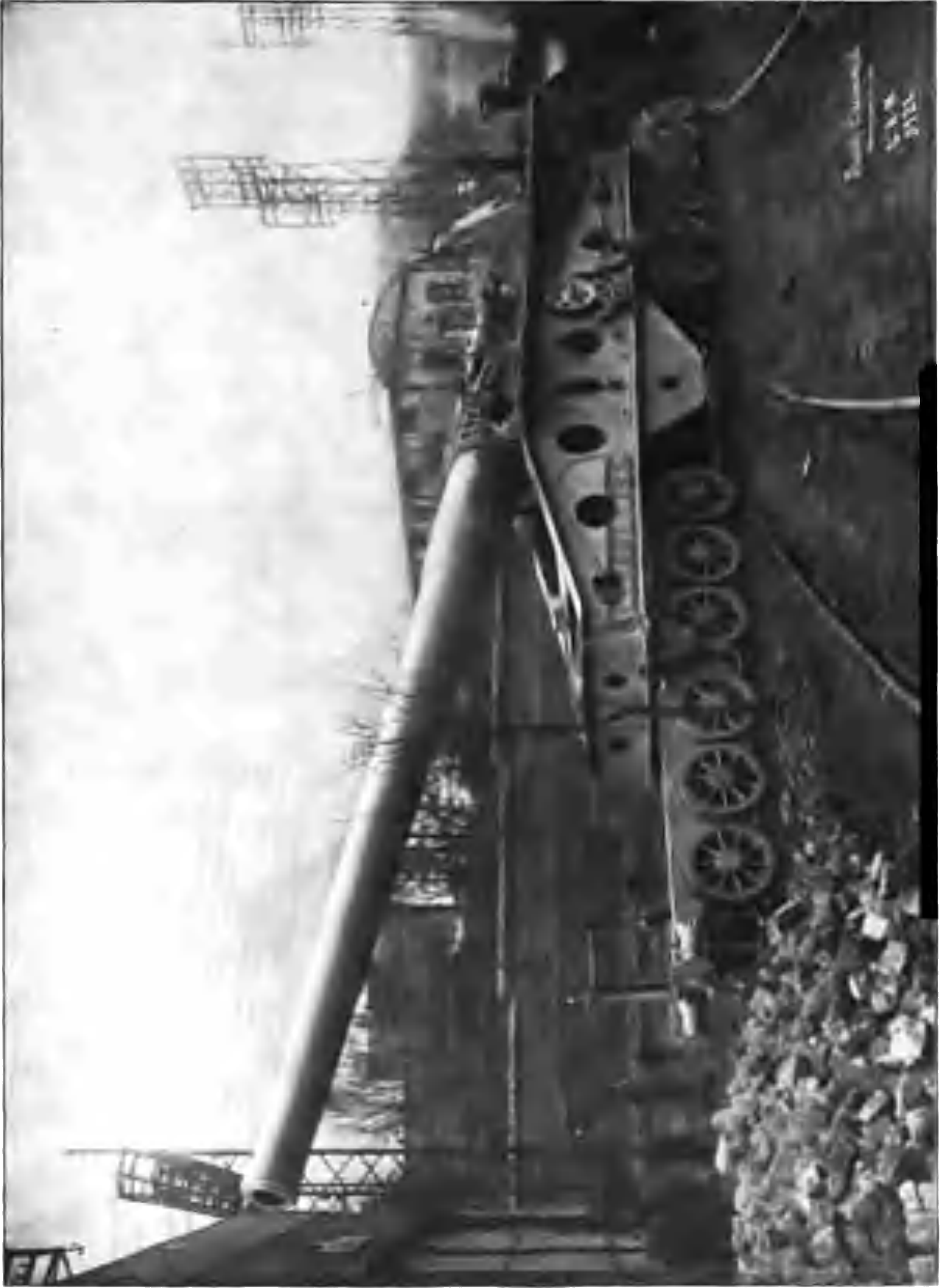
340-MM. FRENCH GUN ON RAILWAY MOUNT.
