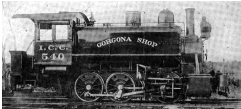
In contrast no. 540 appears to have been reconstructed with a saddle tank, possibly as the works shunter for the shops at Gorgona. The perforated balance weights suggested that this engine began life at a Franco-Belge works, and the wider spacing between the first and second axles imply that it was built to type 27.
