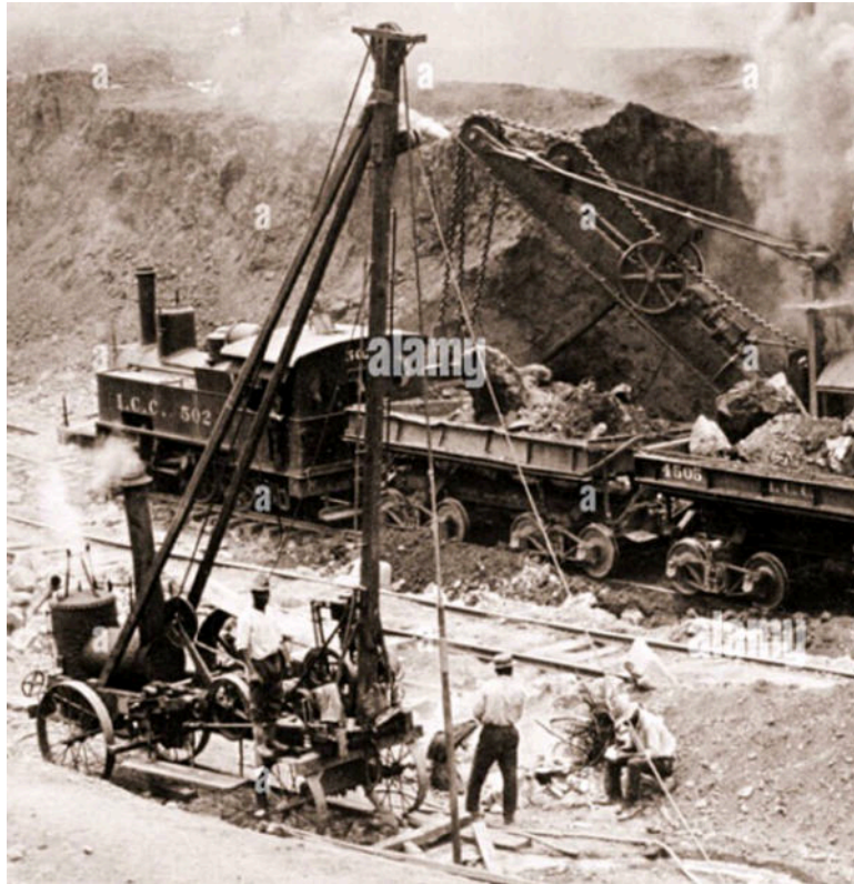
Franco-Belge type 27 no. ICC 502 with a rake of Western dump cars and a steam pile driver in the foreground.
