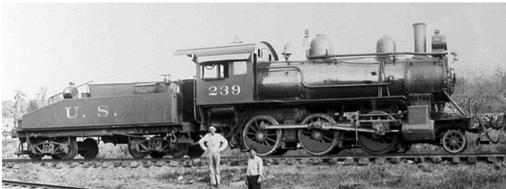
This 201 class loco is seen here more-or-less as built, but with the relatively common addition of a steam take-off pipe leading forward from the dome to enable the powering of a Lidgerwood winch on a wagon immediately in front of the engine.
