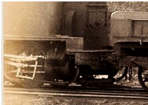
This partial view of a type 88 engine at work with a bucket chain excavator during the 1880s show that the motion protector angle irons were an original or at least a very early fitting.
