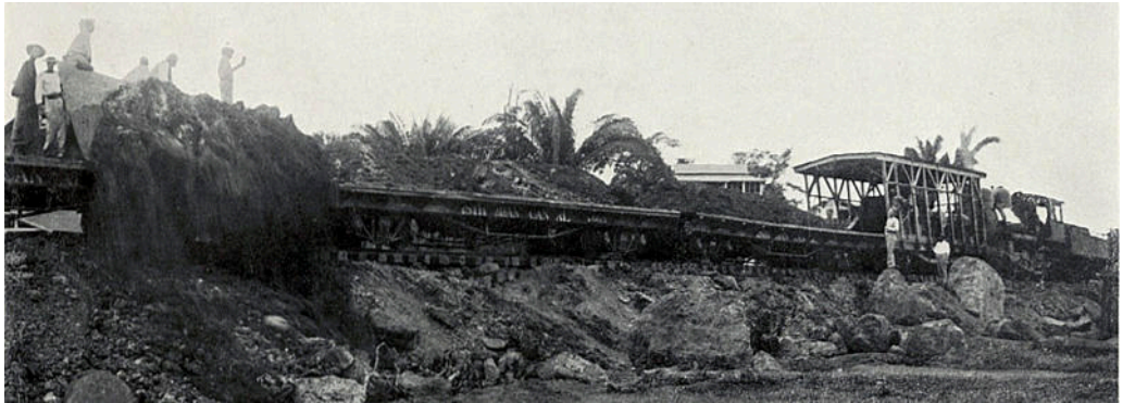
Two views showing the Lidgerwood plough being winched along the train from left to right, with the load of spoil falling alongside the track, from where it will be spread.
