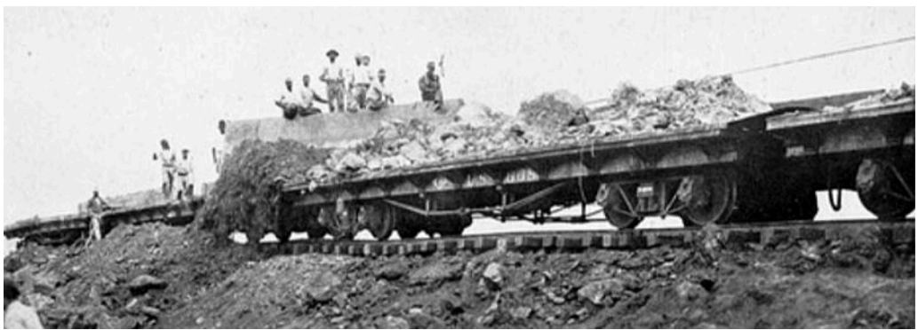
Two views showing the Lidgerwood plough being winched along the train from left to right, with the load of spoil falling alongside the track, from where it will be spread.
