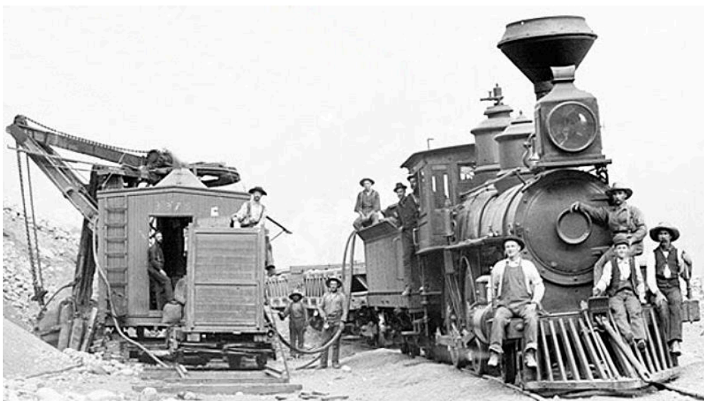
This 4-4-0, seemingly on a canal excavation site, has not yet been identified. It has Rogers / Cooke style domes, a short smokebox like the Rogers engines,
