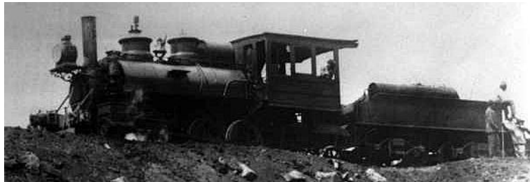
This Rogers 0-6-OST has gained a bogie tender of a very professional looking design, perhaps from one of the 4-4-0 loco types.
