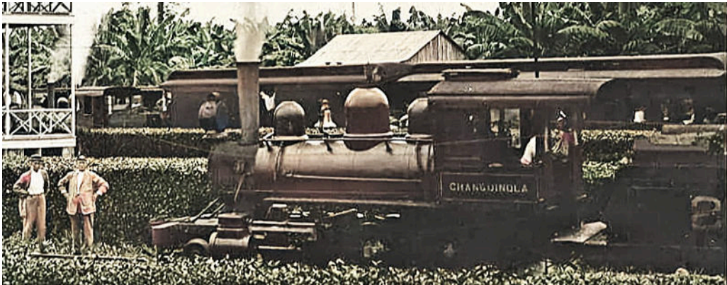
A colourised view of no. 24. You will note that this loco, unlike nos. 18 and 19 seen above, has a rear sand-dome.
